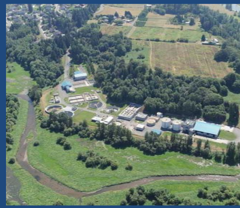
Salmon Creek Treatment Plant
