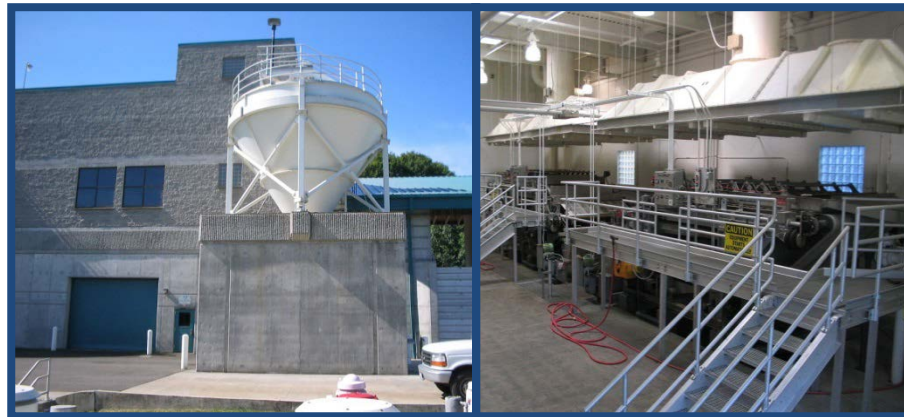
SCTP Solids Processing Center
