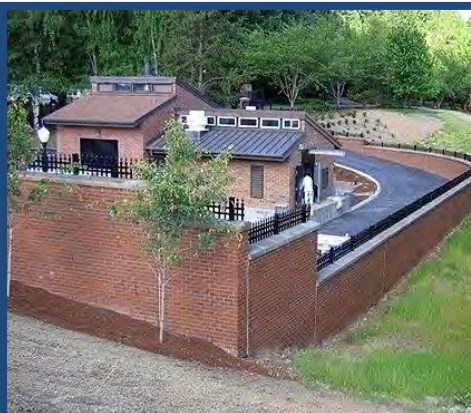
36 th Avenue Pump Station
