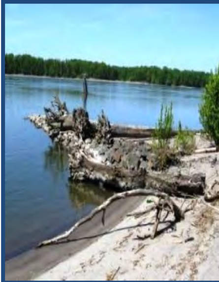
Existing Outfall Installation Low Water
