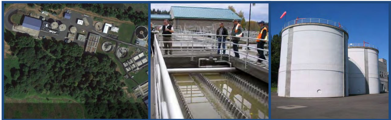
Salmon Creek Treatment Plant Aerial
