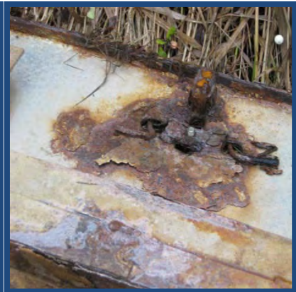
Vault Corrosion
