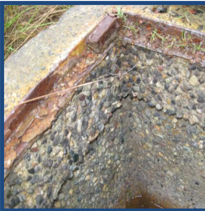
Vault Corrosion
