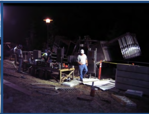
Existing UV System Expansion During Phase 4
