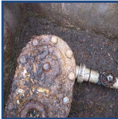
Valve Corrosion
