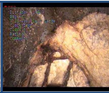
CCTV Image of the Interceptor
