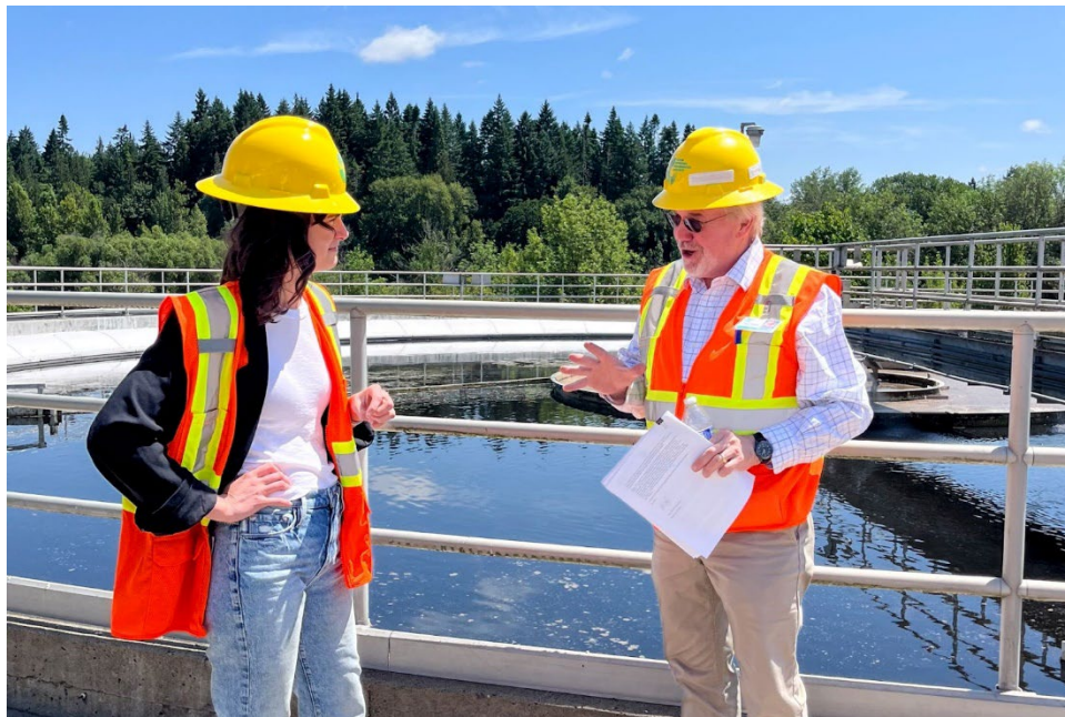
Rep. Gluesenkamp Perez visits the Salmon Creek Wastewater Treatment Plant.
