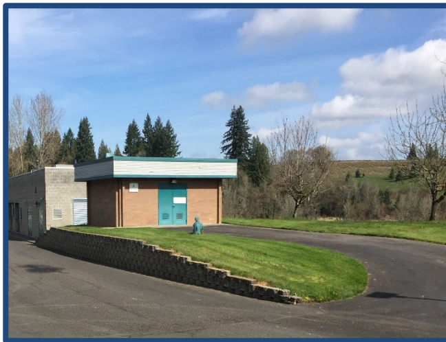
Existing SCTP Well House
