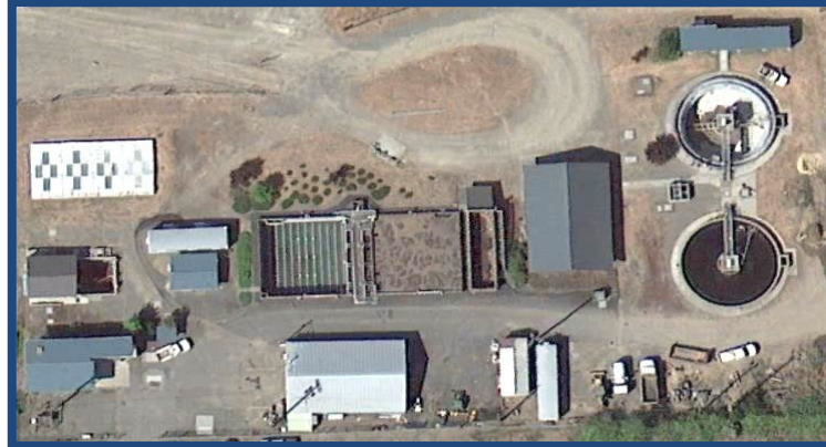
Ridgefield Treatment Plant Site
