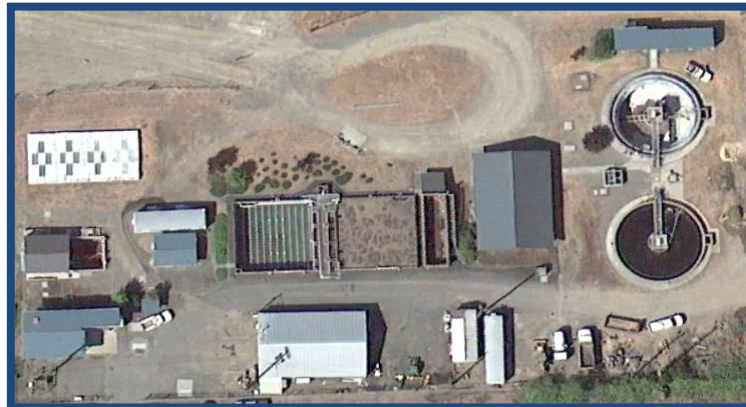
Ridgefield Treatment Plant Site
