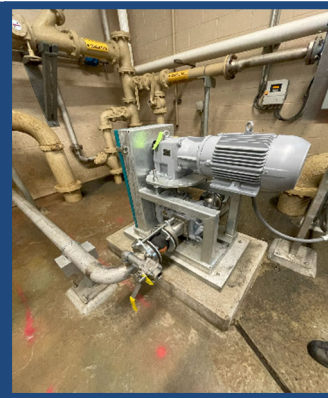
Example Rotary Lobe Style Pump
