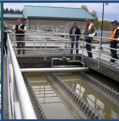
Existing Primary Clarifier
