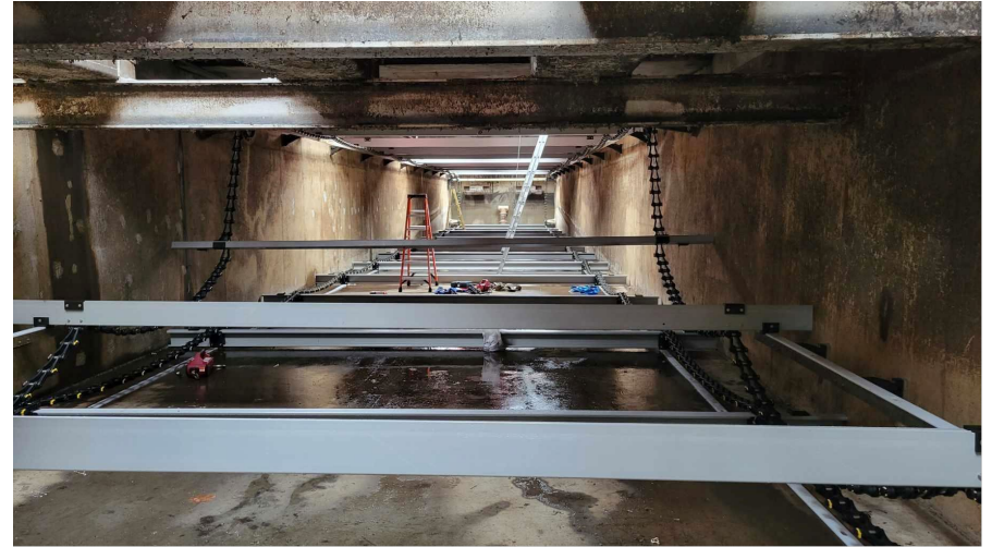
New flights and chain during installation.
