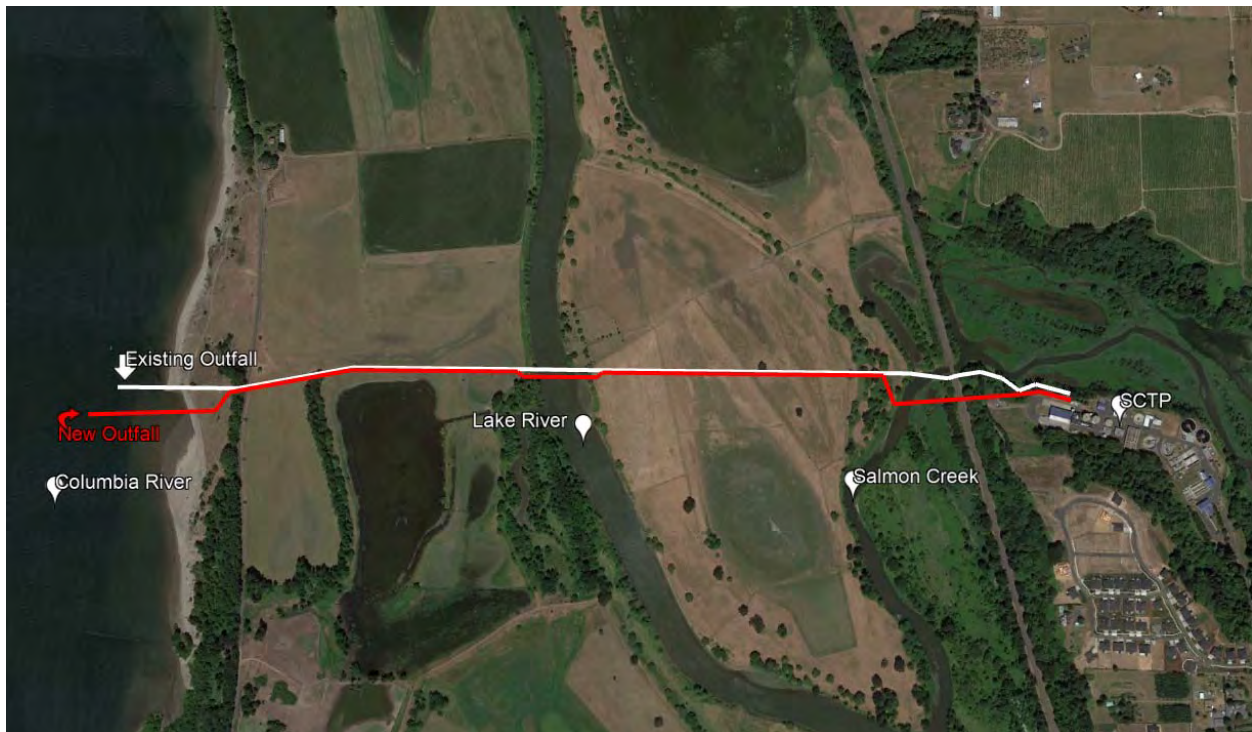
Figure 2-1. Overview of Salmon Creek Treatment Plant, Effluent Pipeline, and Outfall Location on the Columbia River at River Mile 96
