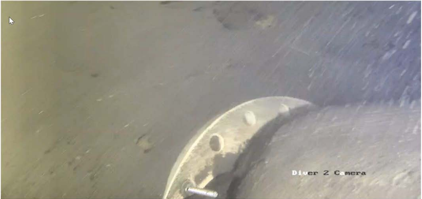
Figure 8 - Break away bolt diffuser #10.
