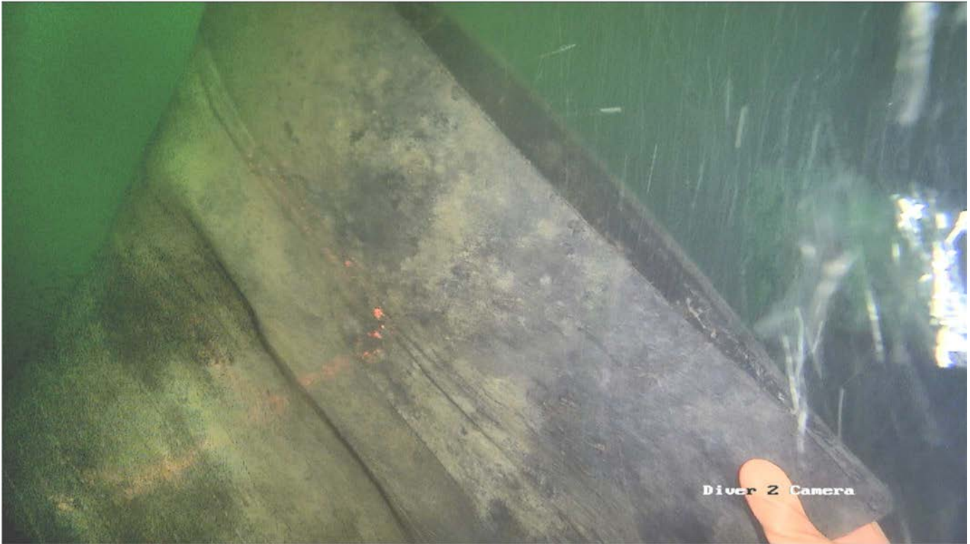
Figure 4 - All 10 diffusers were unobstructed.
