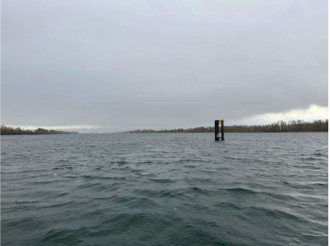
Figure 3 - Salmon Creek outfall dolphin with a buoy on #6 diffuser.
