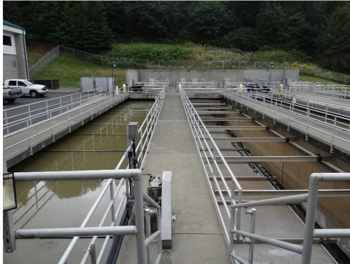
Picture 4-1: Primary Clarifiers
