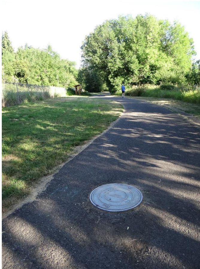
Picture 4-9: Salmon Creek Interceptor Trail Manhole
